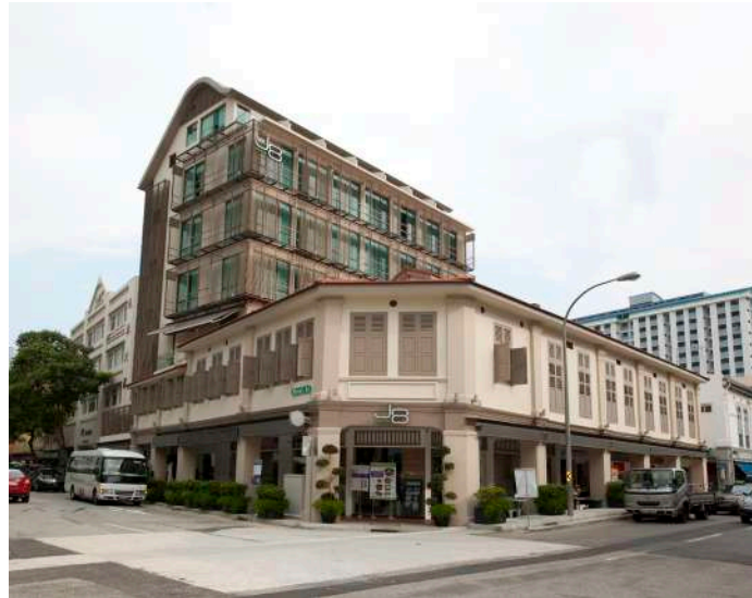
Integration of five Transitional-Style shophouses with new six-storey tower to form a strong streetblock
